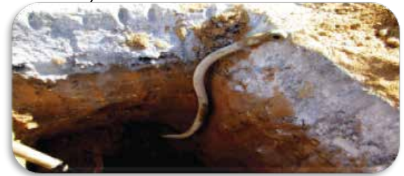
FIGURE I: Lead Service Line
