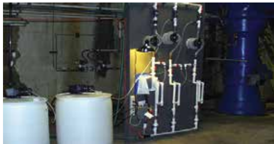
FIGURE I: Corrosion Control Study
