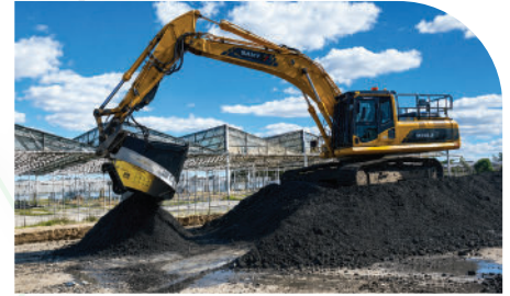
Excavator with Screening Bucket
