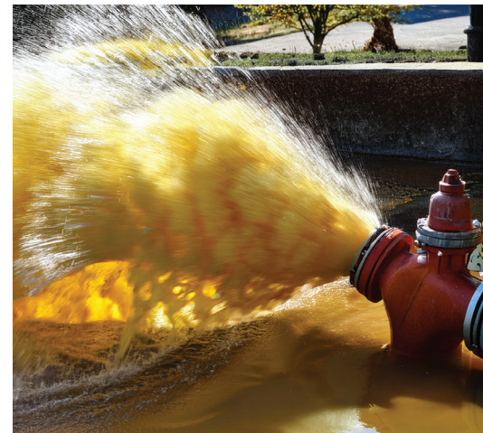
Hydrant Flushing Due to Color Issues
