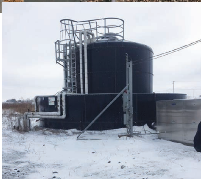
Above: Landfill open cell with electrical panel for leachate discharge. Right: An above ground storage tank containing leachate from the landfill with closure on right side housing the lift station pump. Images courtesy of Carus Corporation.
