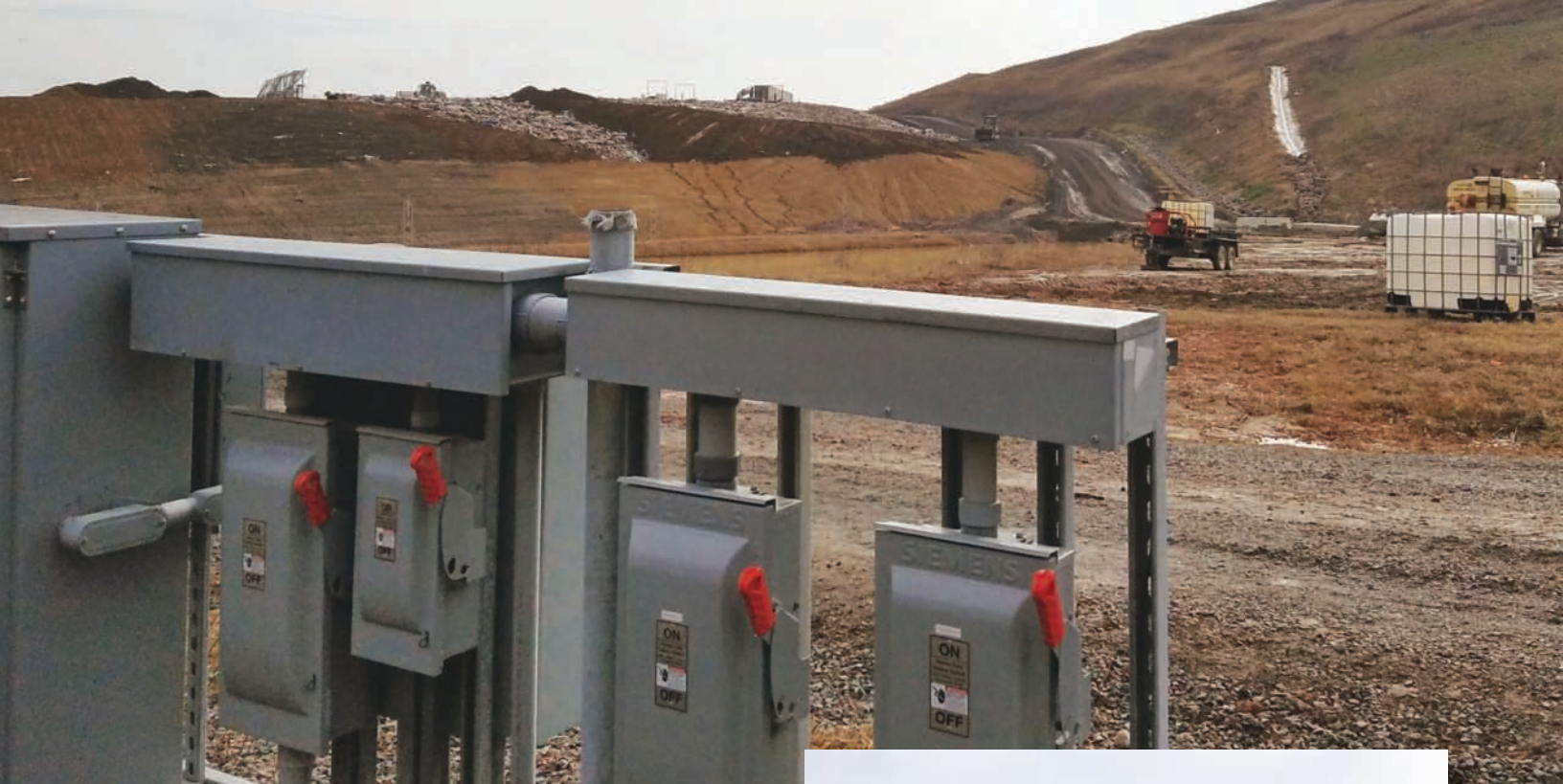
Above: Landfill open cell with electrical panel for leachate discharge. Right: An above ground storage tank containing leachate from the landfill with closure on right side housing the lift station pump. Images courtesy of Carus Corporation.
