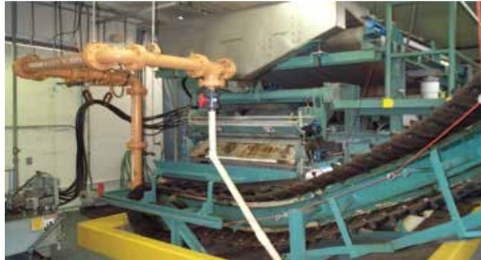
Figure 1: Belt Filter Press at Milan (IL) Wastewater Treatment Plant.
