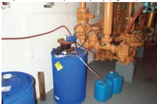
Figure 3: CARUSOL delivery system (drum and feed pump).
