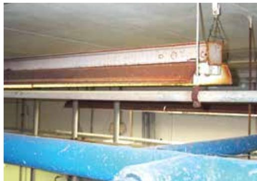
Figure 2: Surface corrosion in dewatering room due to hydrogen sulfide.
